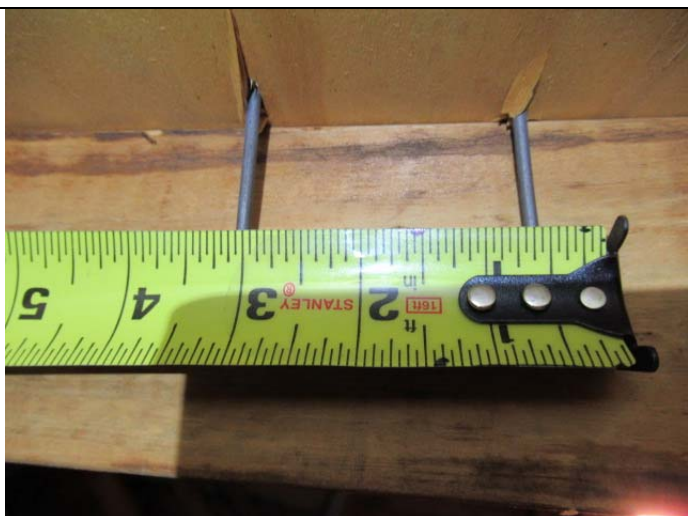
Roof deck attachment
