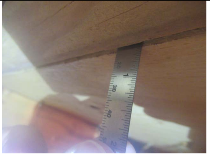
Roof deck thickness
