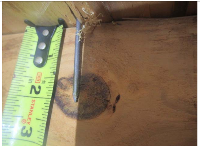
Roof deck attachment
