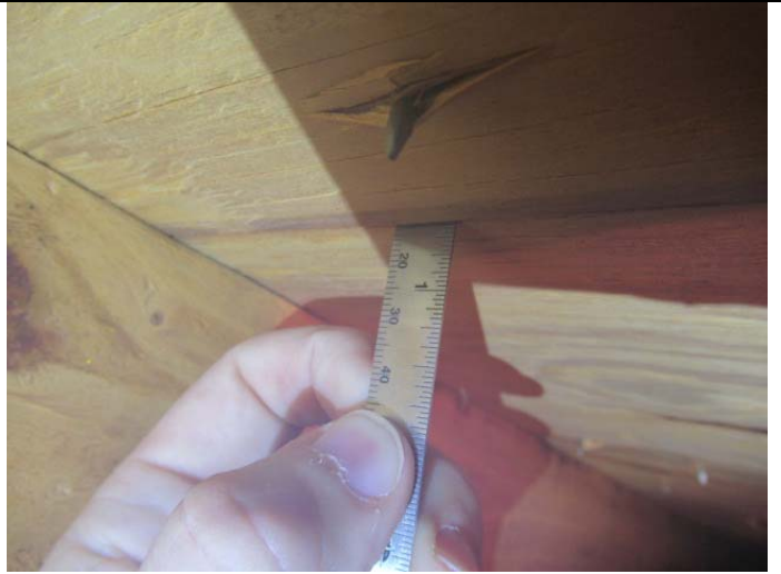
Roof deck thickness
