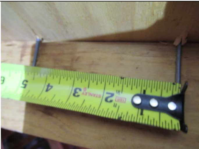
Roof deck attachment
