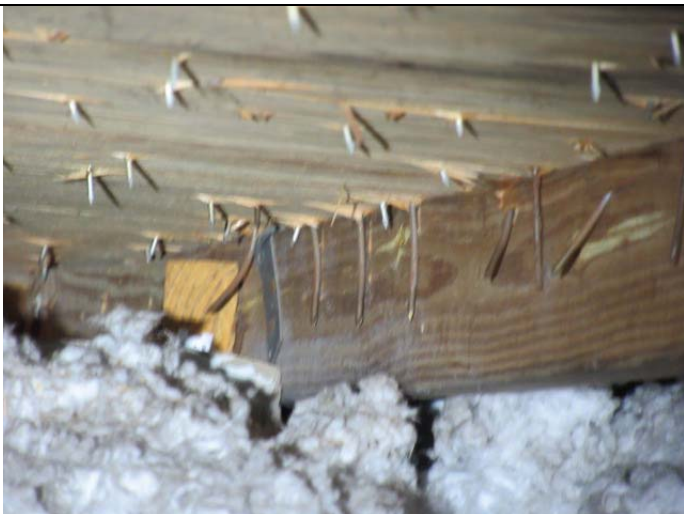
Roof to wall attachment
