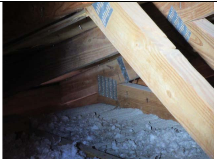
Roof to wall attachment
