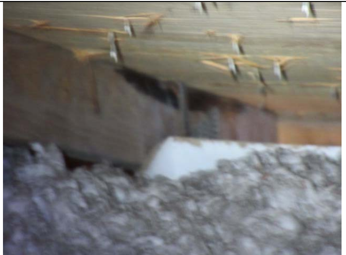
Roof to wall attachment
