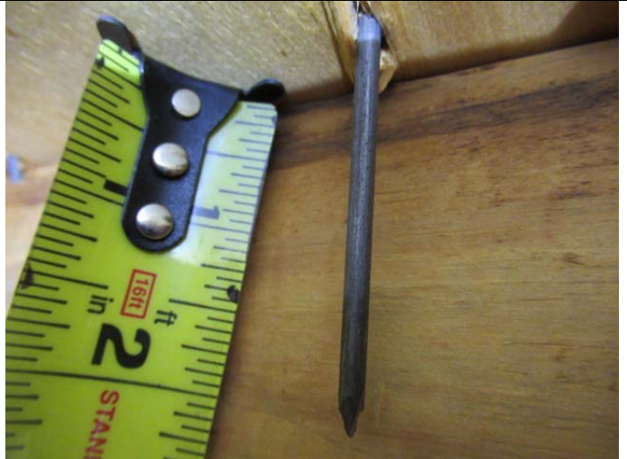
Roof deck attachment
