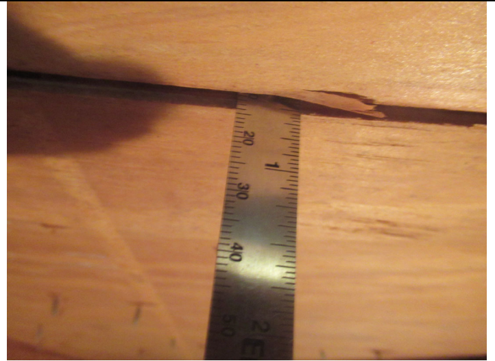
Roof deck thickness
