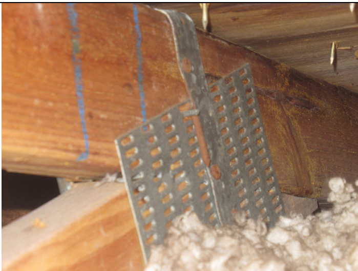
Roof to wall attachment
