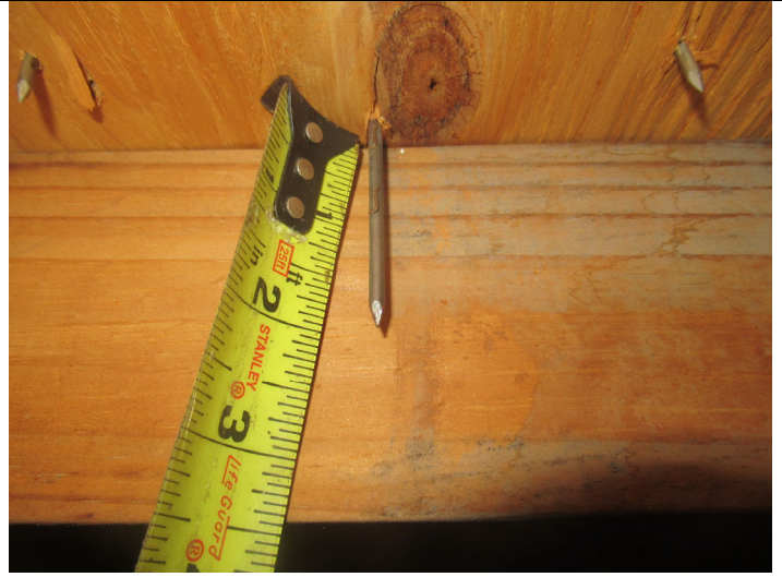
Roof deck attachment
