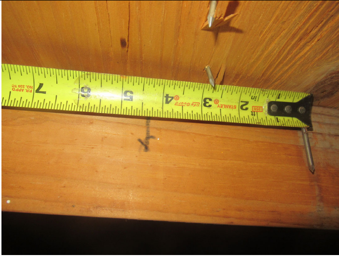
Roof deck attachment
