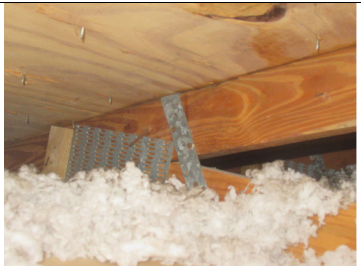
Roof to wall attachment
