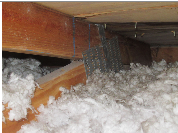
Roof to wall attachment
