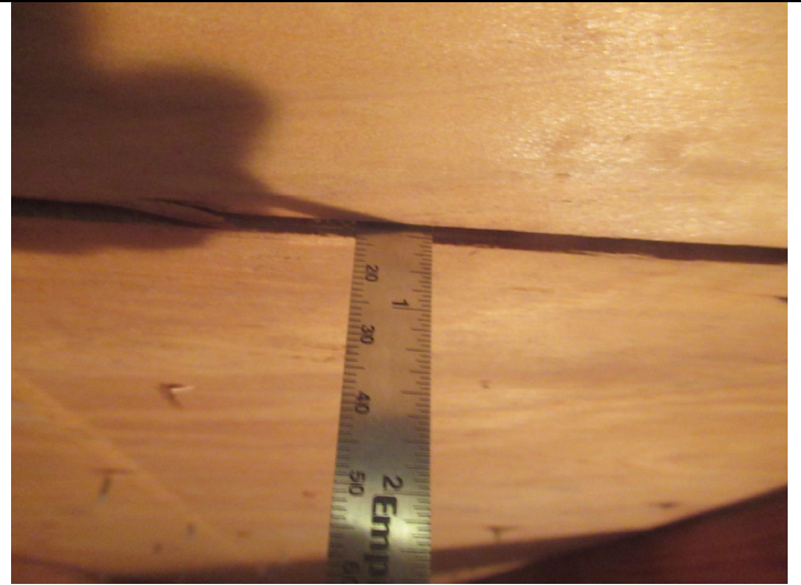
Roof deck thickness
