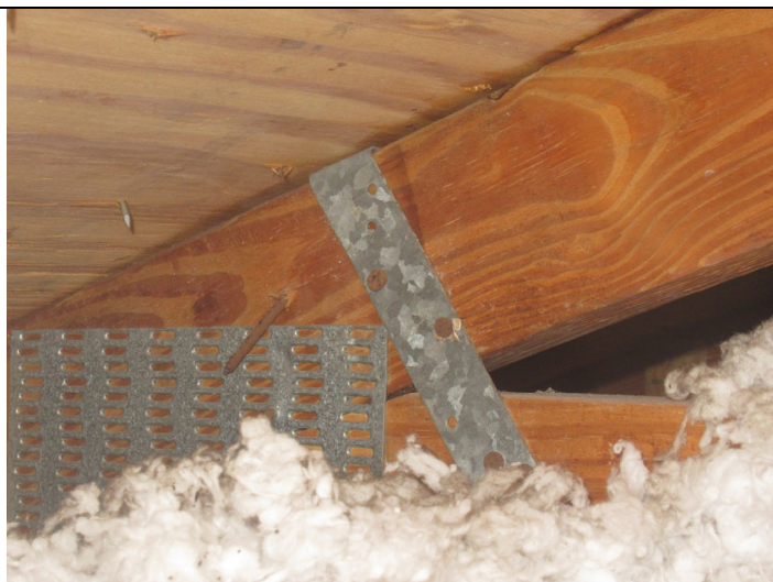
Roof to wall attachment
