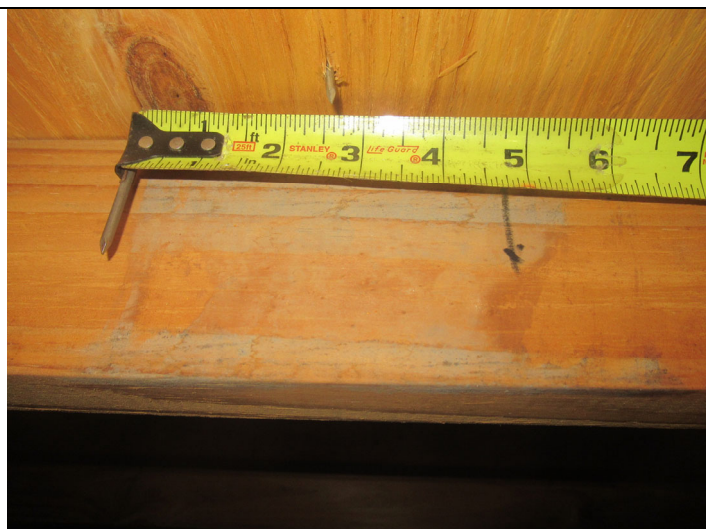
Roof deck attachment
