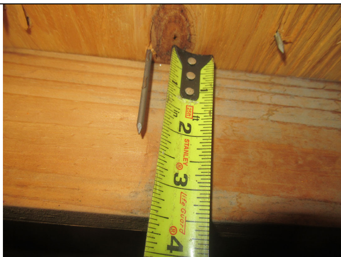
Roof deck attachment
